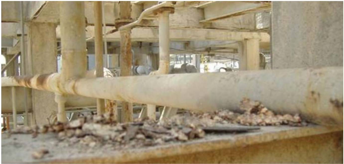
Figure 4. 2" Dummy Support Leg Welded to 3" Pipe at a 90° Angle
